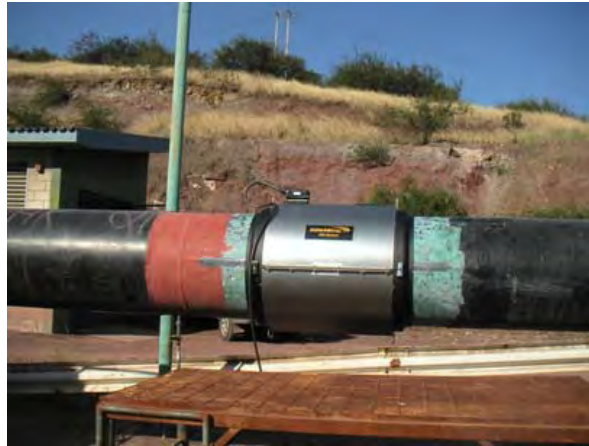
Figure 18 SONARtrac installation on a high pressure pipeline
