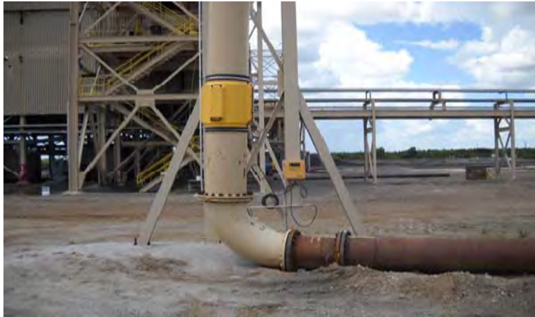
Figure 5 Down-leg installation at Wingate
