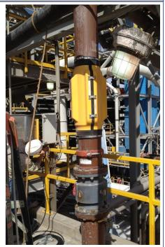
compatible with clamp-on ultrasonic flowmeters, and invasive electromagnetic flow meters require special metal flanges be attached to the fiberglass pipe, adding cost. *SONARtrac* meters solve these costly problems.
