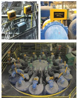
Figure 5 Installed CYCLONEtrac OSM System with transmitter and junction box (upper left picture), sensor head (upper right picture), and a completely instrumented hydrocyclone battery (bottom picture)
