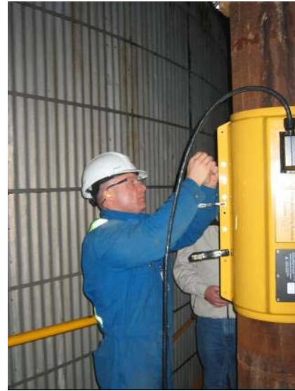
Figure 15: Installation of Sonar-based flow meter on 16 inch commercial bitumen froth line
