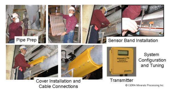
Figure 1 - Installation procedure from (top-left) pipe preparation through cleaning and light sanding of pipe to (top-middle and top-right) mounting of the flexible, lightweight sensor band to (bottom-left) installation of the sensor cover and to (bottom-middle and bottom-right) connection of sensor cover to transmitter via water tight cable
