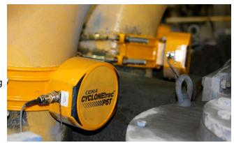
The CYCLONEtrac PST system consists of individual sensor assemblies mounted to hydrocyclone overflow pipes, junction boxes, and a control room computer (or virtual server). The sensor assembly is made up of a ruggedized sensor element that is in contact with the overflow stream and an integrated electronics package that is protected by a sealed metal enclosure. The sensor assembly is wired to the junction box located near the hydrocyclone battery. The junction box receives 100-240 VAC
