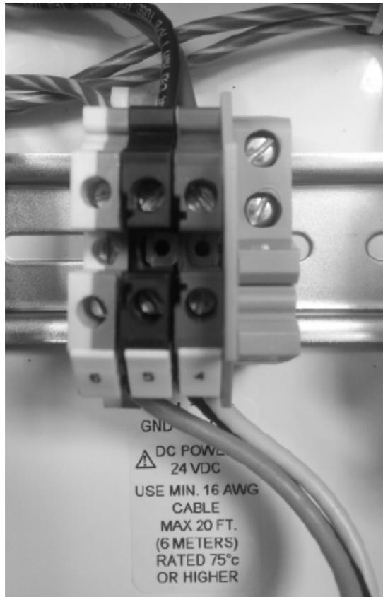
**Figure 16: DC Power Connection, Power Entry Box**
