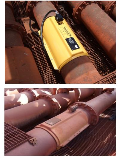
*SONARtrac* Process Measurement Systems, sonar-based clamp-on technology for the most challenging processes.
