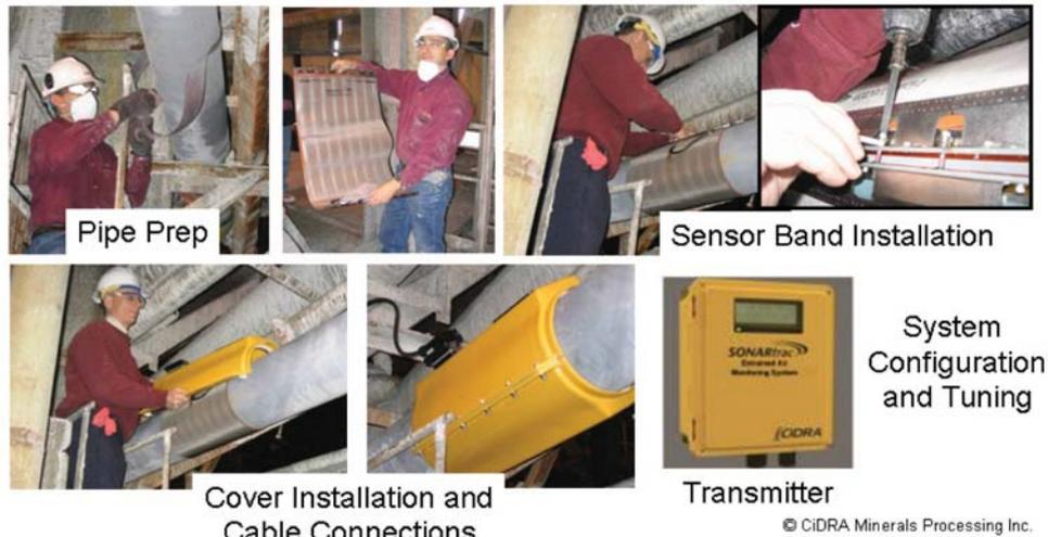
**Figure 1. Installation procedure (from top left to bottom right: pipe preparation through cleaning and light sanding of pipe; mounting of the flexible, lightweight sensor band; installation of the sensor cover; and connection of sensor cover to transmitter via the watertight cable**
