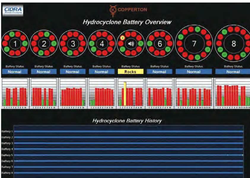
Figure 7—Screen capture of control room computer monitor.
