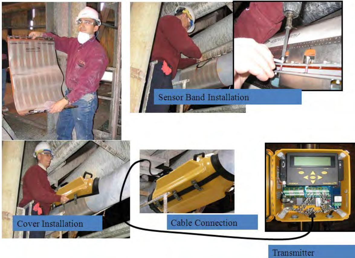
**Figure 2. Installation procedure from (top left) pipe preparation through cleaning and light sanding of pipe; (top middle and top right) mounting of the flexible, lightweight sensor band; (bottom left) installation of the sensor cover; and (bottom middle and bottom right) connection of sensor cover to transmitter via watertight cable**
