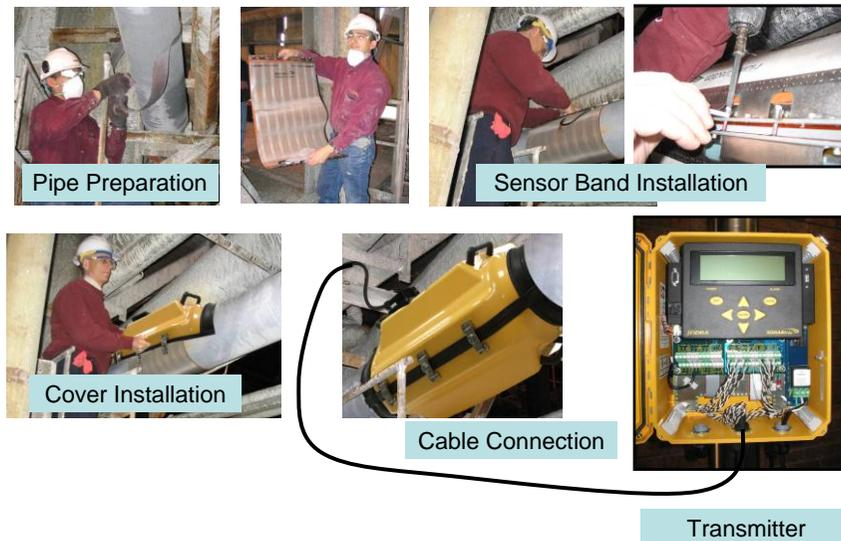
Figure 1 - Installation procedure from (top-left) pipe preparation through cleaning and light sanding of pipe to (top-middle and top-right) mounting of the flexible, lightweight sensor band to (bottom-left) installation of the sensor cover and to (bottom-middle and bottom-right) connection of sensor cover to transmitter via water tight cable
