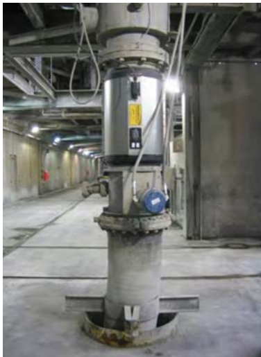
Figure 3: Passive Sonar Flow and Entrained Air Meter
