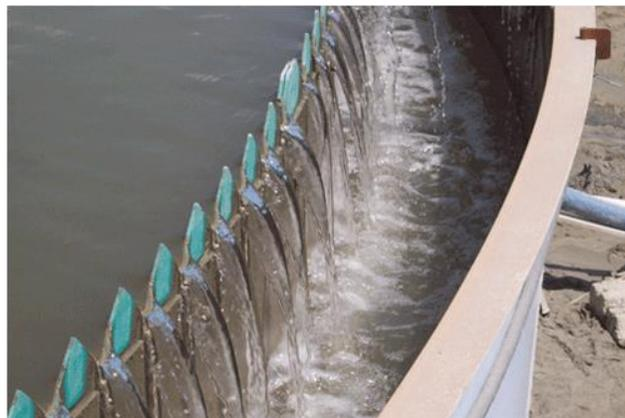
Figure 10 Clear Water Exit Channel
